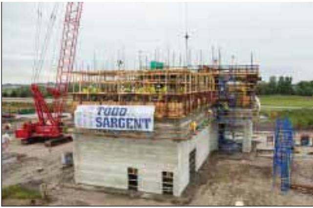
Todd & Sargent's construction crews worked 24 hours a day for 4-1/2 days to pour cement for the 100-foot-tall feed mill tower. Photo courtesy of Iowa State University.
